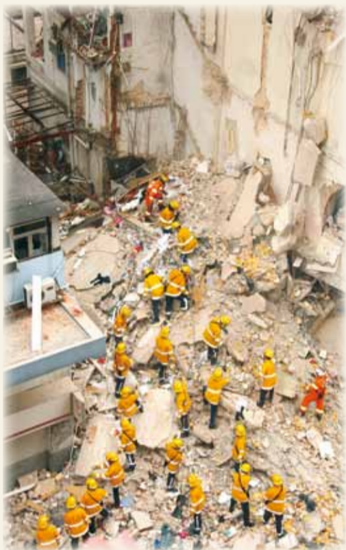
• 救援人員在瓦礫中搜救被困人士 F.S. personnel conducting search and rescue after the collapse of the building
